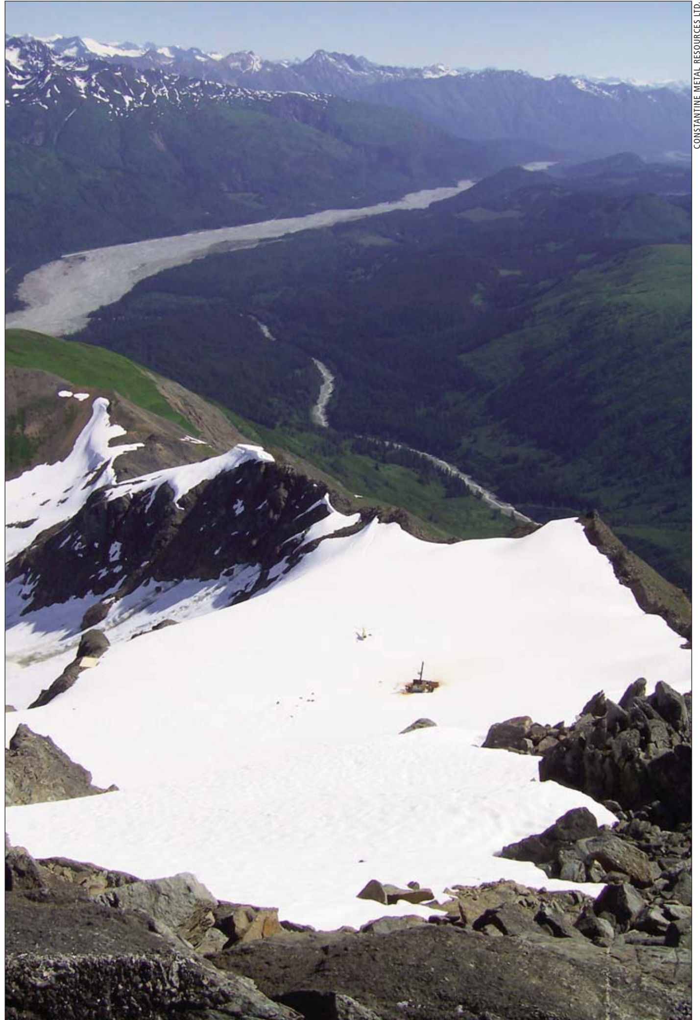
A drill cuts through snowpack into the RW Zone at Constantine Metal Resources' Palmer property in Southeast Alaska. CMR 10-35 cut 7.1 meters averaging 2.10 percent copper, 1.52 percent zinc, 0.18 grams per metric ton gold and 16.8 g/t silver.
